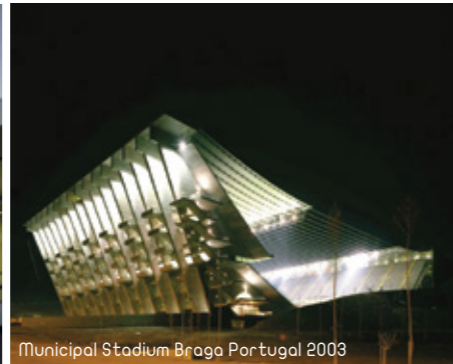
Municipal Stadium Braga Portugal 2003
