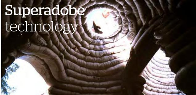
The system employs the timeless forms of arches, domes and vaults to create single and double-curvature shell structures that are both strong and aesthetically pleasing. While these load-bearing or compression forms refer to the ancient mudbrick architecture of the Middle East, the use of barbed wire as a tensile element alludes to the portable tensile
