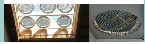
The **SunBeamer** skylight is a clever and surprisingly simple daylighting solution that directs sunlight exactly where you need it most. Developed by SunCentral, the sun-tracking circular skylight uses rotating mirrors to shoot beams of light deep within a building.
